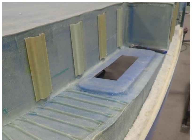
Figure 22. Flotation foam on the sides of the deck
